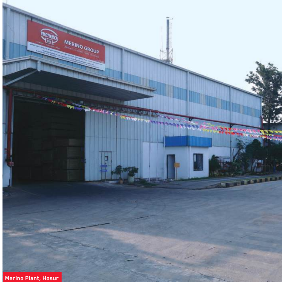
Merino Plant, Hosur
