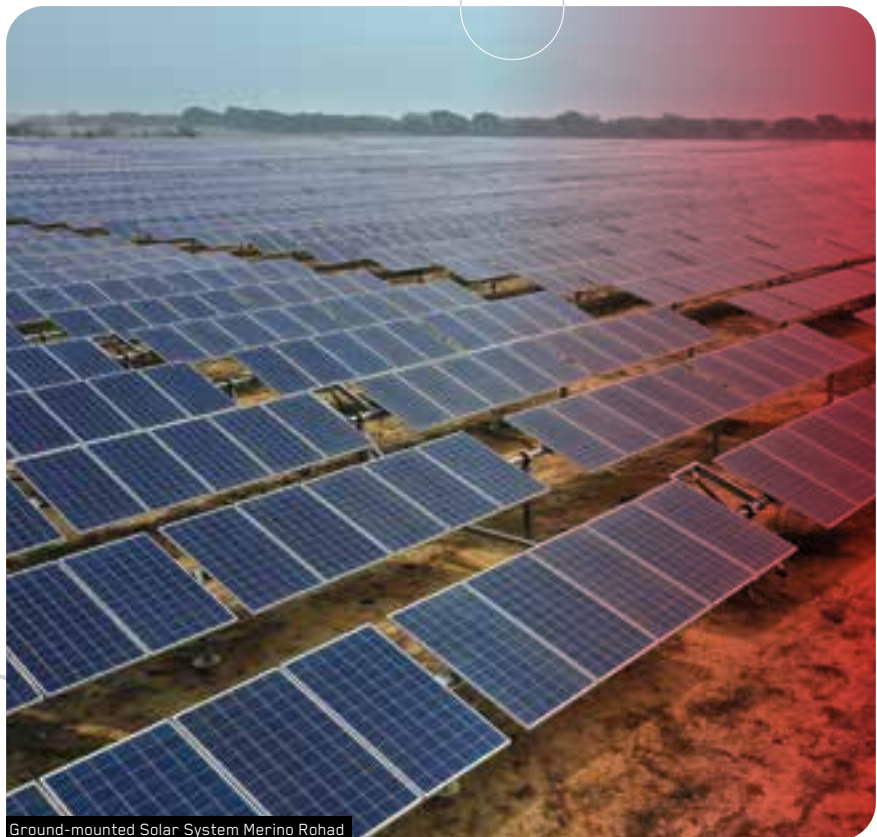
Ground-mounted Solar System Merino Rohad
