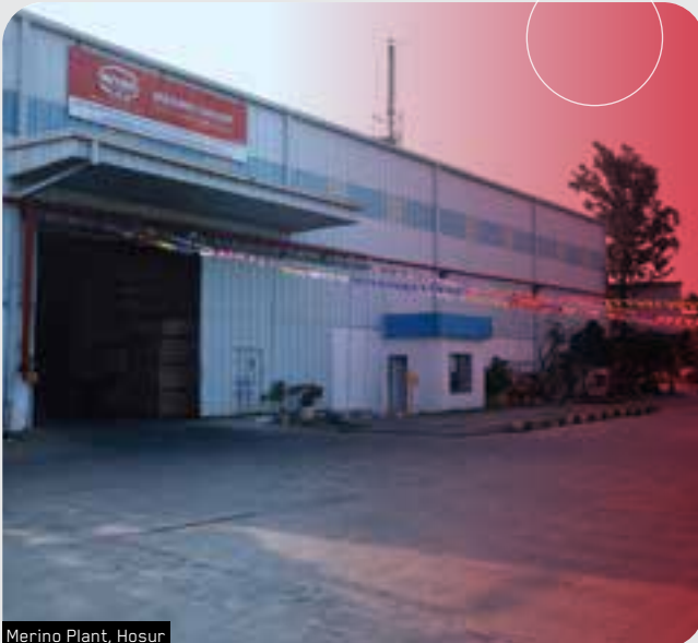
Merino Plant, Hosur
