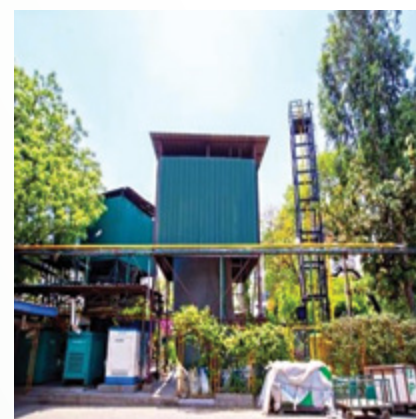
^ Biogas System from In-House Organic Wastes, Generated around 1,87, 316 SCM Unit in FY 2024-25
